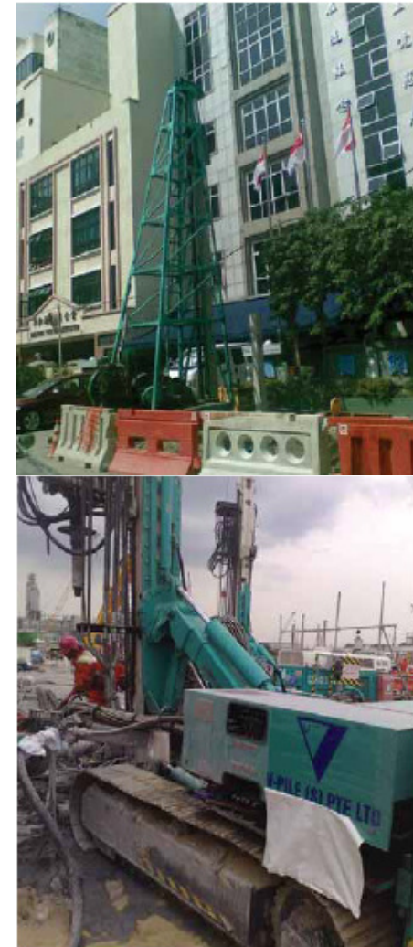
V-Pile piling works in Singapore
